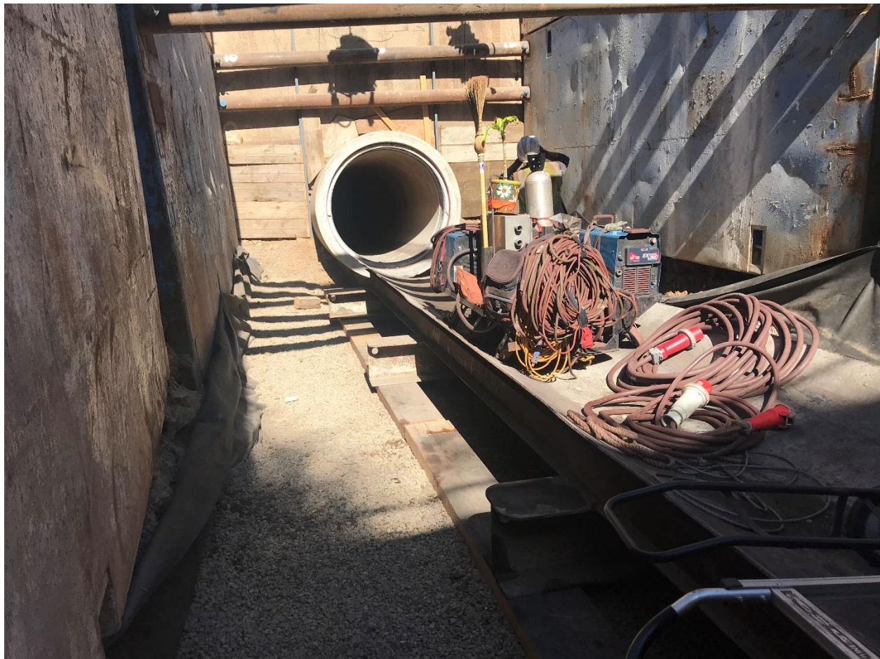
Figure 37. Relining pipeline at Lake Murray (Source: Cell-Crete Corporation)
