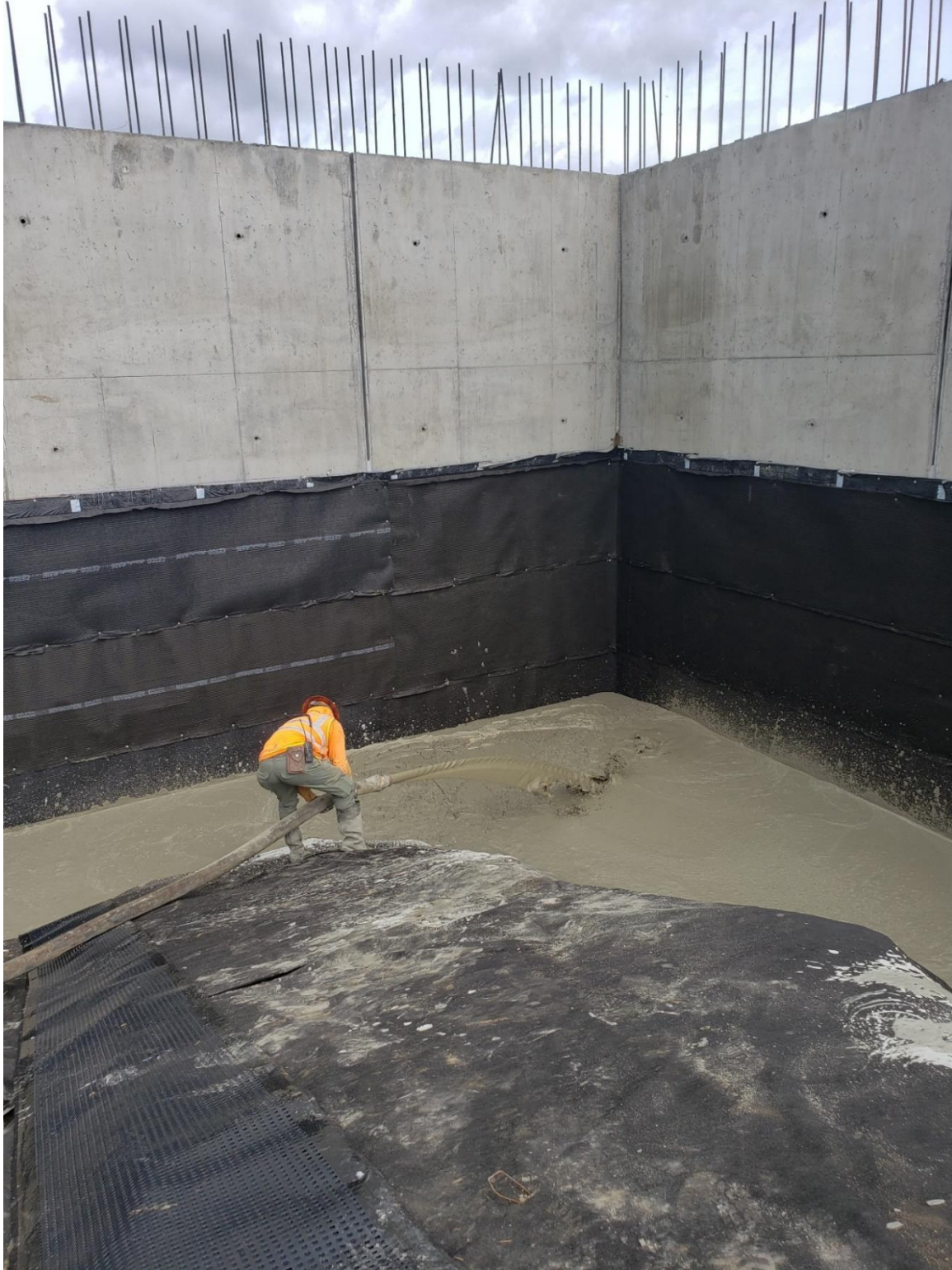
Figure 46 a and b – Overview of the LCC placement at the LCG Columbia Storage project. (Source: Source- Cell-Crete Corporation)
