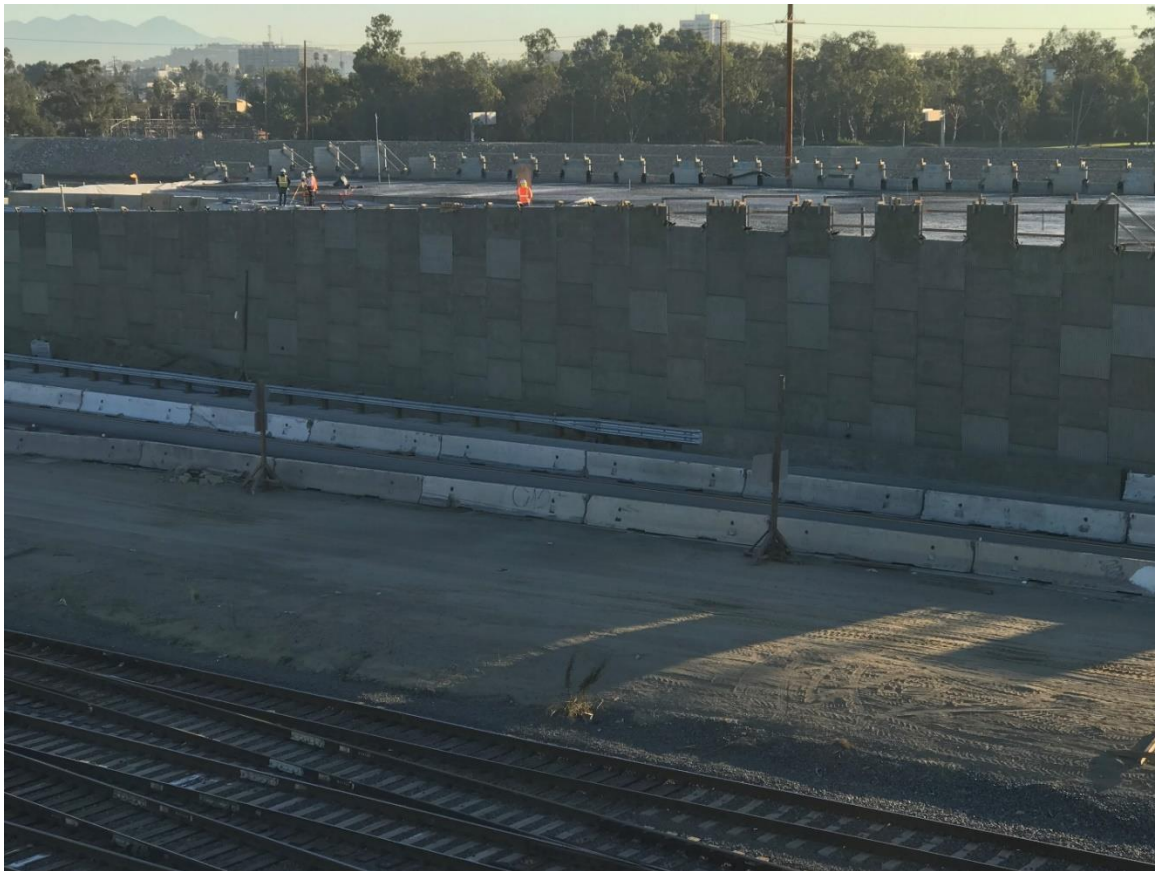
Figure 40 LCC MSE wall at Gerard Desmond Bridge project (Source: Cell-Crete Corporation)
