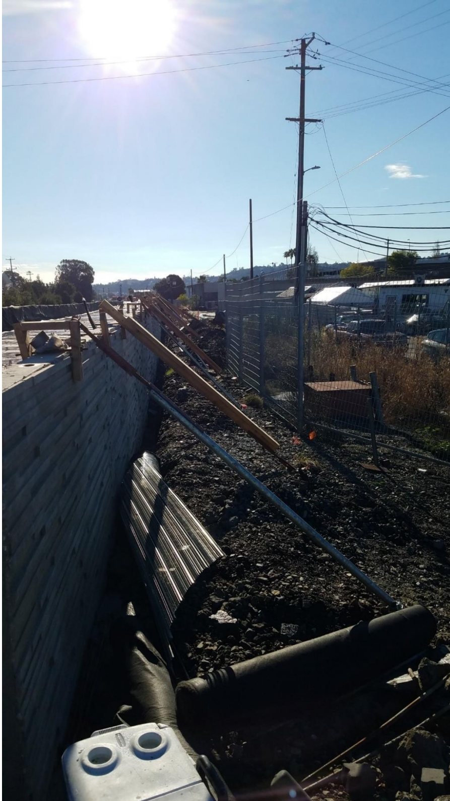
Figure 48 Overview of 25 th Avenue Grade Separation project (Source: Throop Lightweight Fill)
