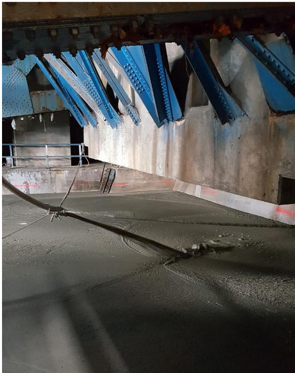
Figure 43: LCC material used in the Roosevelt Avenue Bridge (Source: Aerix Industries)
