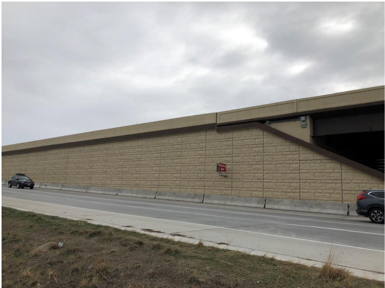
Figure 44 MSE Wall constructed for the SR-154 project (Source: Gerhart Cole Inc.)
