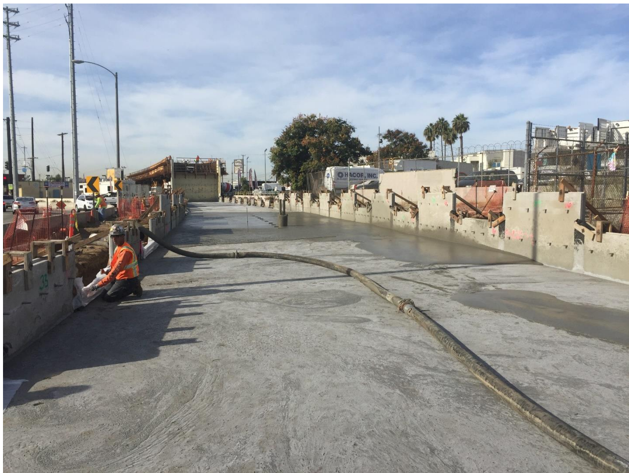
Figure 39 LCC material used for the Crenshaw Corridor/ LAX Transit project (Source: cell-Crete Corporation)
