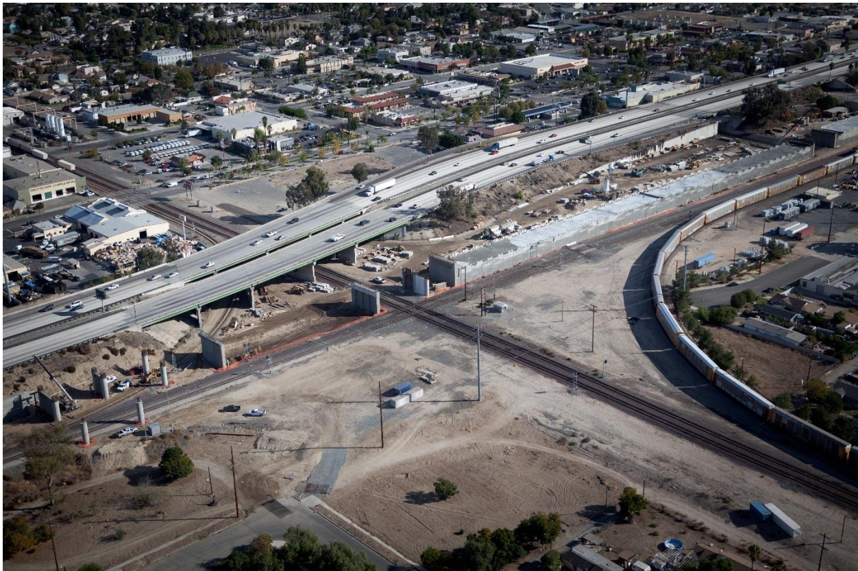
Figure 41 LCC MSE wall constructed at Colton Crossing (Source: Cell-Crete Corporation).
