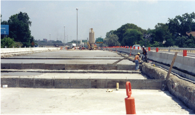
Figure 1.2. Lightweight road subbases and fills (Ohio)
