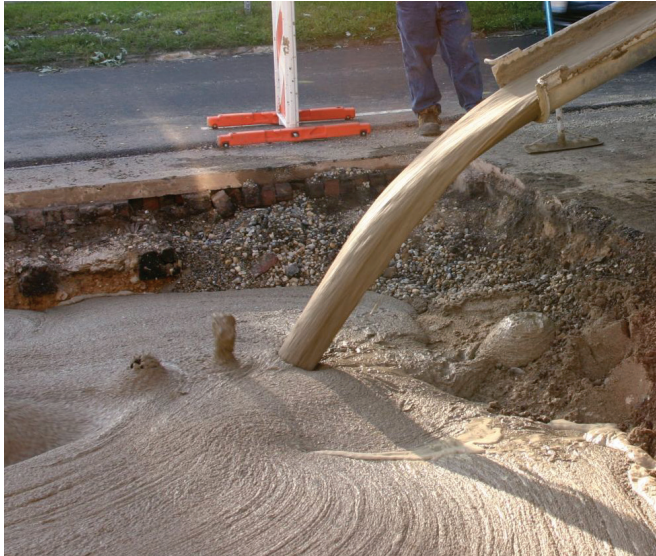
Figure 1.13. Controlled density fill
