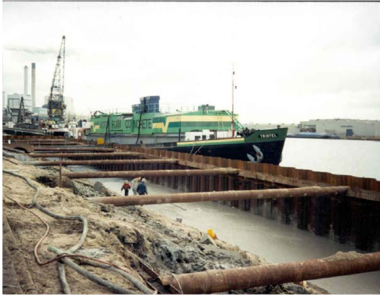
Figure 3. Picture of Lightweight Fill Project in The Netherlands.
