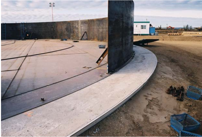
Figure 2. Cellular Concrete used for insulation below above ground storage tanks.
